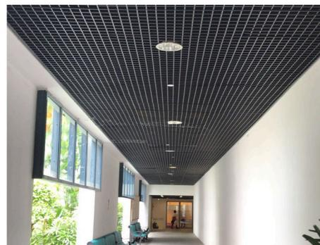
Aluminum cell ceiling system see through ceiling give one a spacious feeling and the ceiling elegant and distinctive looks. Its exposed surface is powder coated with non-toxic polyester paint in RAL or Oxyplast colour code.
